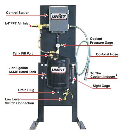
\*NOTE: For Thru-Spindle applications there are separate air and coolant lines.
